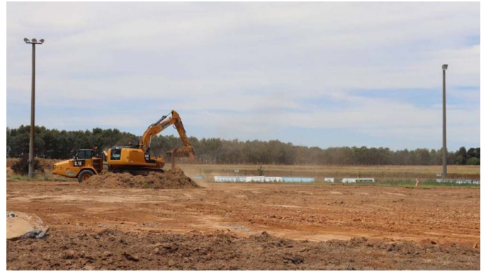
Lead remediation by excavation in Australia. Photo Credit: Turfmate Editor, AU
